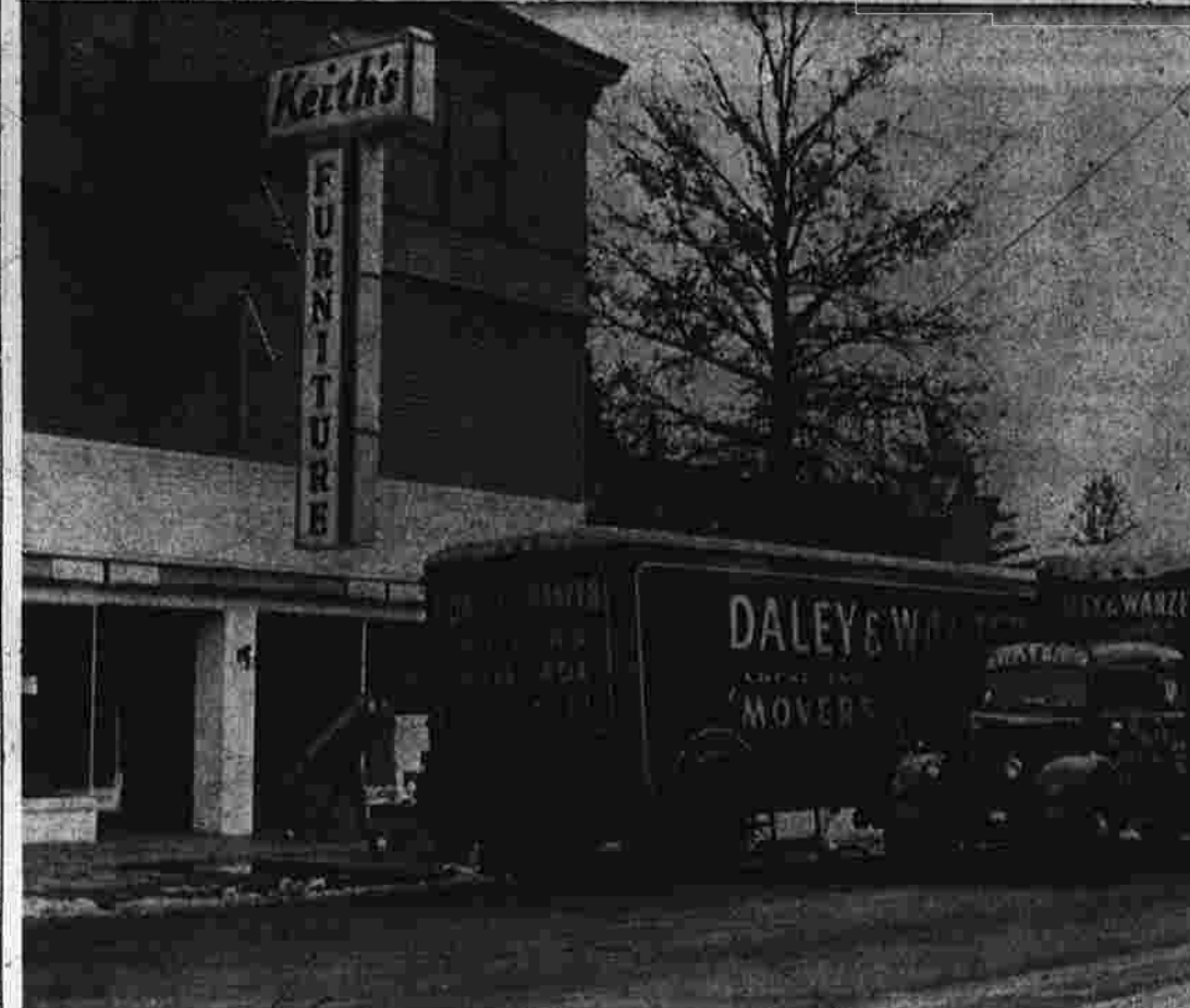
Damaged Stock Leaves Keith's Furniture Two large motor vans from Massachusetts load up with water damaged furniture from G. E. Keith Furniture store's recent fire. More than $20,000 worth of stock was sold for salvage to a Massachusetts discount bargain center. Shipments of new furniture are on the way and the firm expects to be ready for Christmas shopping next week. It was reported today. (Herald photo by Orlan).
